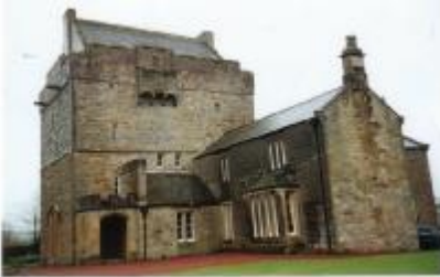
The Pele, or Peel Tower, at the village of Elsdon.
