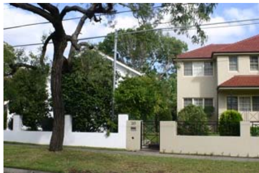
An example of a power pole on a property which is similar to that proposed by the Eruv.
